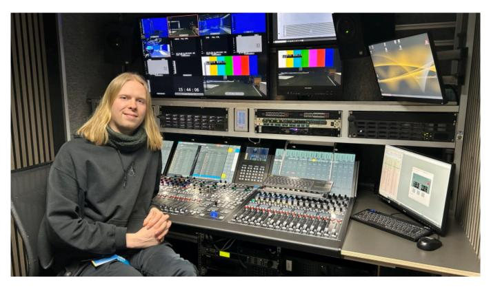
Studio Berlin has completed a comprehensive modernization of its OB truck Ü2, integrating cutting-edge Audio-over-IP (AoIP) technology from Lawo. At the heart of this upgrade is a 48-fader mc²56 MKIII console, replacing the previous mc²66 mixing desk. Additionally, A\_stage units have been implemented as I/O devices, along with the mc² DSP App, providing 256 DSP channels. The existing Lawo VSM system has been expanded to optimize control over the IP-based broadcast infrastructure.
