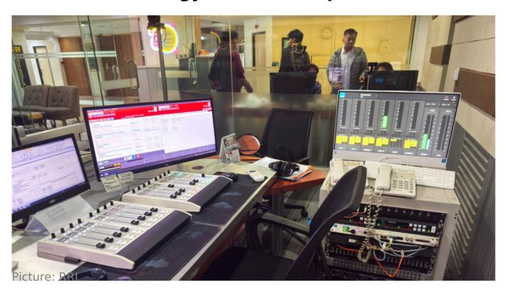
Radio Republik Indonesia (RRI), Indonesia's national public broadcaster, has modernized its studios with state-of-the-art Lawo solutions, installing three 14-fader crystal mixing consoles and a Power Core router. Ordered in October 2024 and completed by December, this upgrade enhances operational efficiency, streamlines workflows, and establishes in two steps a future-proof, fully IP-based broadcast infrastructure.
