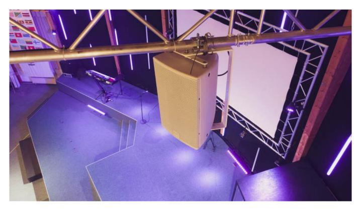
After comparative listening, the decision was finally made in favour of Martin Audio. Since the church building is a rotunda with a gallery, the sound system was divided into sections. The area in front of the stage is the largest area to be covered (with two CDD12s). The upper tier, which uses a glass pane as a parapet, was covered with two CDD10 loudspeakers. The difficulty was to hit the glass surfaces as little as possible, in order to avoid reflections.
