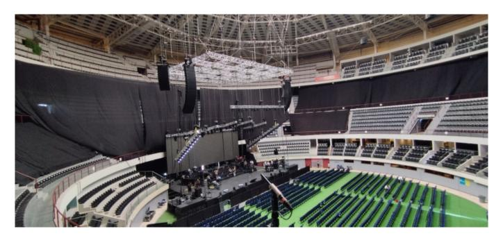
The full deployment at the GNP Acapulco Arena included 16 WPL per side for the main hang, run off iKON amps (in 2-box resolution), and eight MLA per side for outfill,. Subs comprised 24 SXH218 in an Inverted stack array. By designing it in a cardioid arc, it was able to cover 120° and provide a homogeneous and coherent coverage from the first rows to the farthest, right at the top of the venue. So complete was the coverage that only minimal front fill coverage was required.
