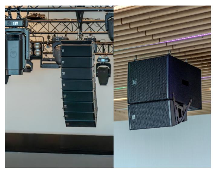
Complementing this is a delay of four TORUS T820 8" constant curvature speakers, providing defined 100° by 20° coverage pattern in the meeting areas at the mezzanine level, while four auxiliary CDD-LIVE 12 can be used as infills or outfills as required. Martin Audio's ADORN 5.25" ACS-55T ceiling speakers are set underneath the mezzanine to provide main system delays, or for independent use when this space is separated from the main hall - providing immense versatility.
