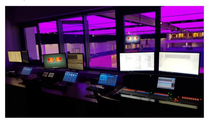
Control for the AFC system is via Yamaha ProVisionaire Touch on iPad, with presets for the different modes making the system very easy to operate.
