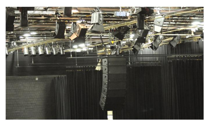
The line array's five top speakers emit at a narrower angle (SEQUENZA 10 N) whilst the two at the bottom emit at a wider angle (SEQUENZA 10 W). If necessary, another three subwoofers (SEQUENZA 10 B with cardioid directional coverage) are used on each side.
