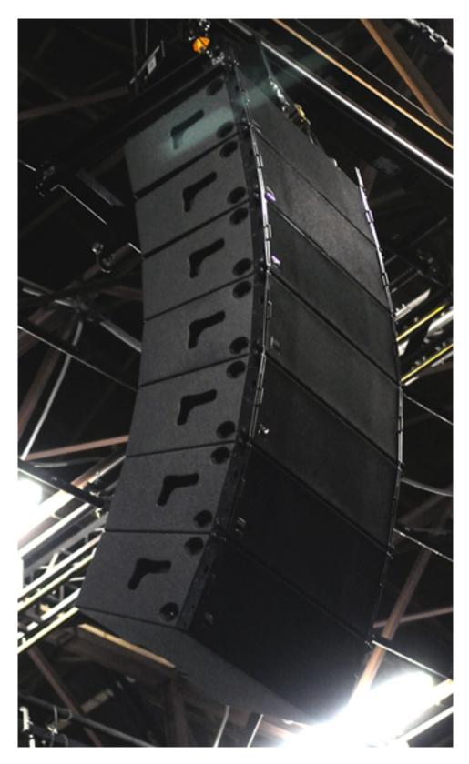
Other speakers in Hall K6 are the two GRAVIS 12 N as nearfills, two CA 1001 as delays and two more CA 1001 as nearfills or monitors etc. The system is supplied by five Kling & Freitag SystemRacks.
